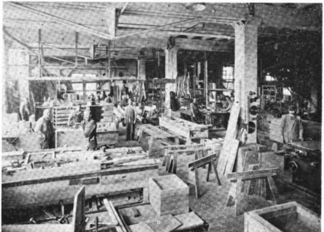
A corner in the well equipped joiner shop of the Skinner & Eddy plant.
