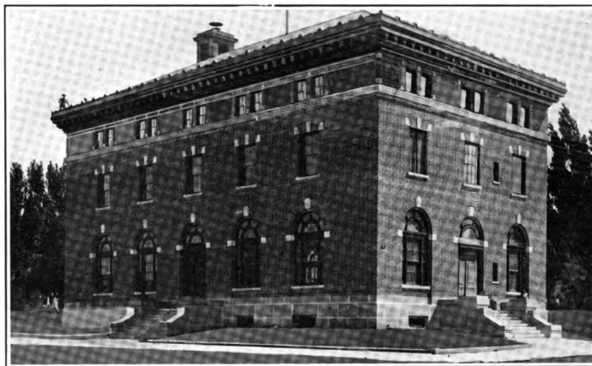
Federal Building, Moscow, Idaho (Tenino Stone)
